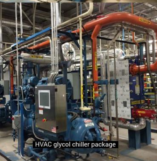
Screw compressor for HVAC glycol chiller
