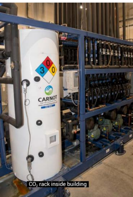
Pipes from CO 2 rack carrying CO 2 gas to roof for condensation
