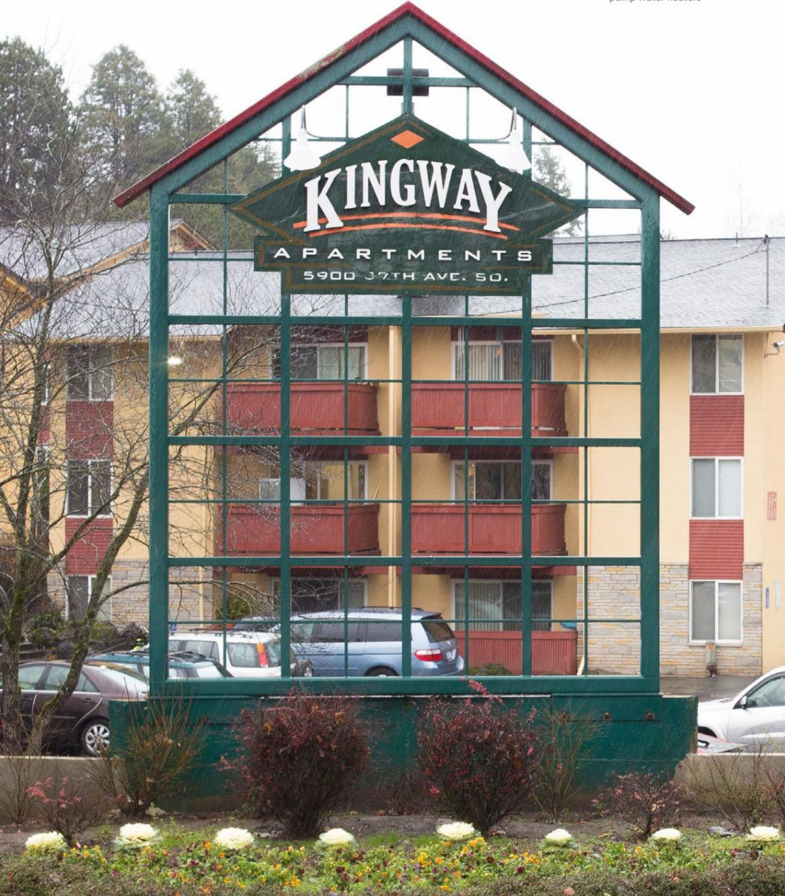
Seattle location of the installation of CO 2 heat pump water heaters
