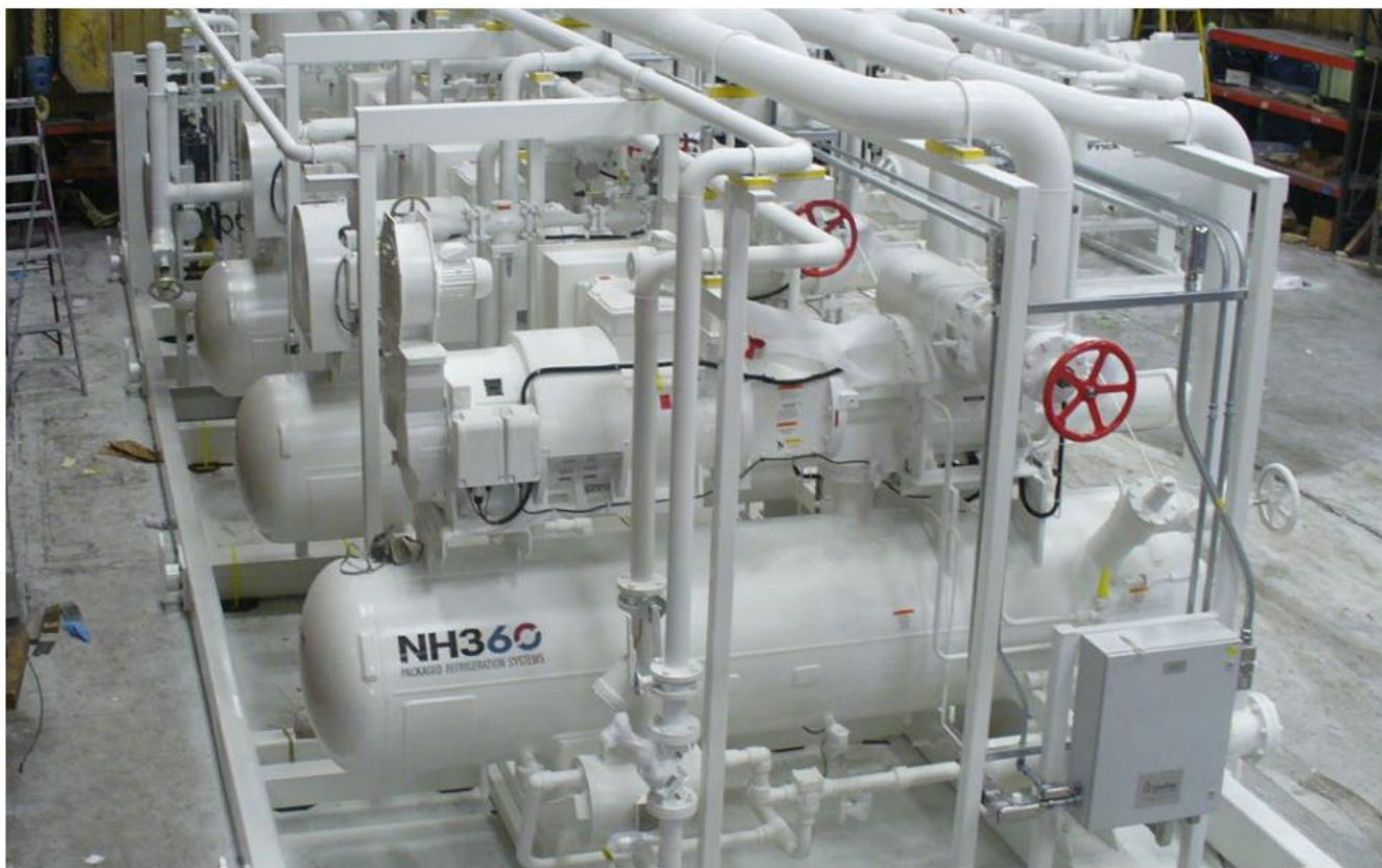
Stellar NH360 packaged low-charge-ammonia system
