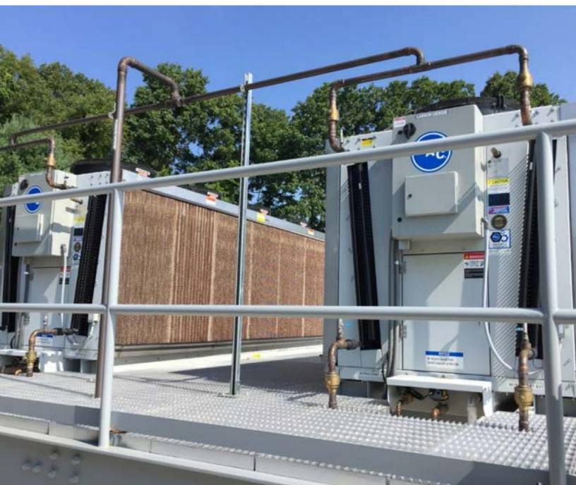
BAC adiabatic condensers used with Weis Markets’ transcritical system
