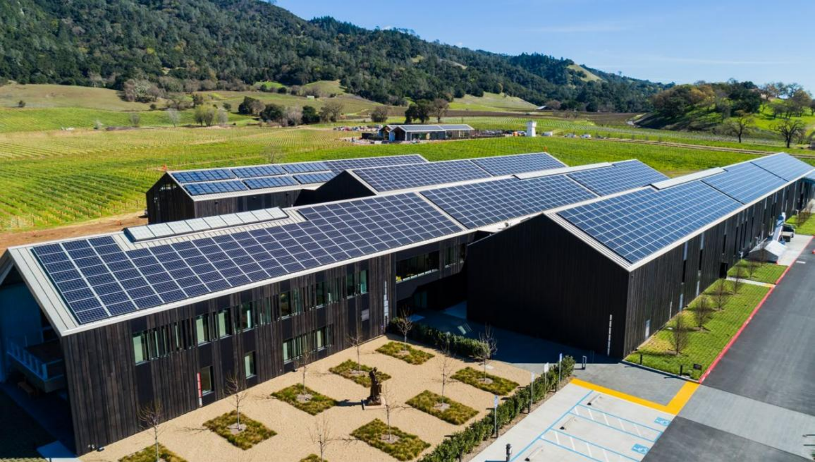
Silver Oak's winery in Healdsburg, Calif., which heats water with solar energy and CO 2 heat pumps
