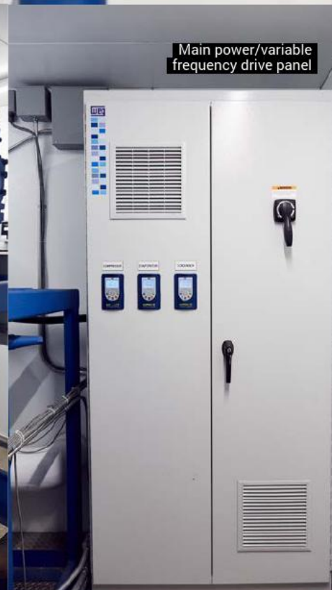
RPM display and control modules for variable frequency drive
