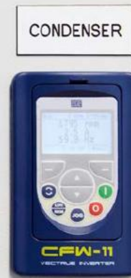
RPM display and control modules for variable frequency drive
