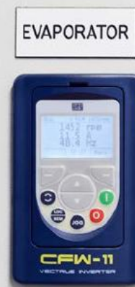
RPM display and control modules for variable frequency drive
