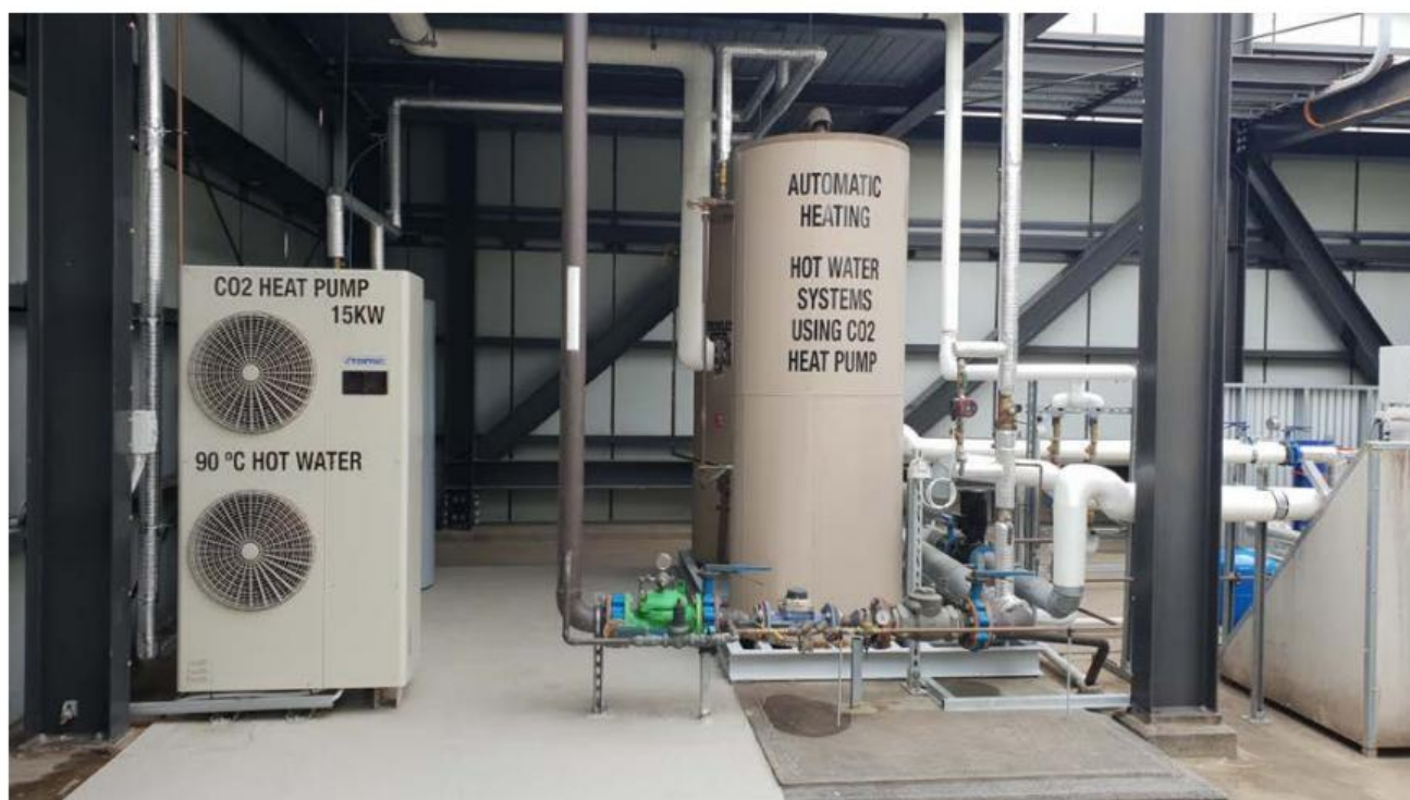
Itomic Eco-Cute 15kW High Temperature CO 2 Heat Pump
