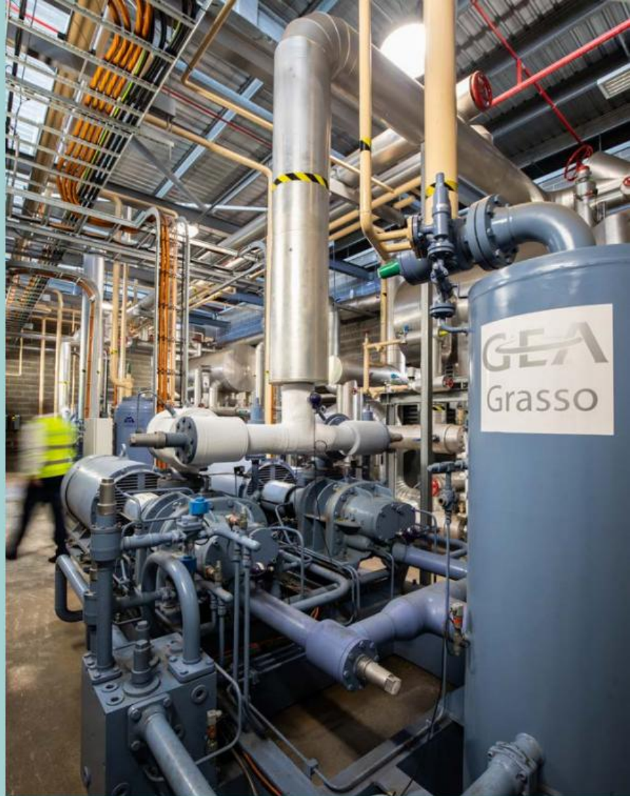
GEA Duo Pack compressor package for propylene glycol chilling duty.
