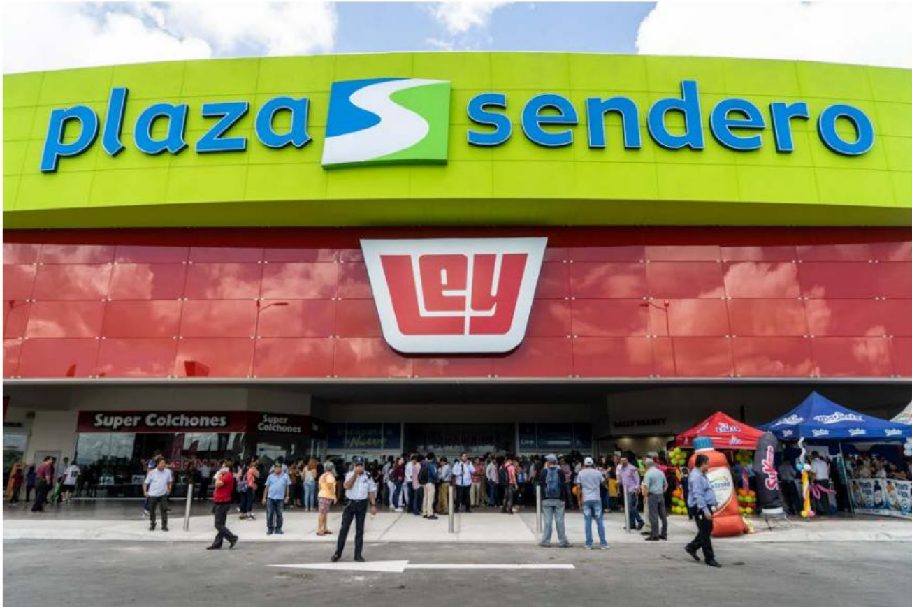
Casa Ley's pilot CO 2 transcritical store in Culiacán, which opened in August.
