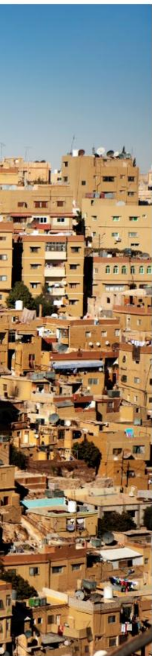
Amman, home to the first CO 2 transcritical supermarket in the Middle East.
