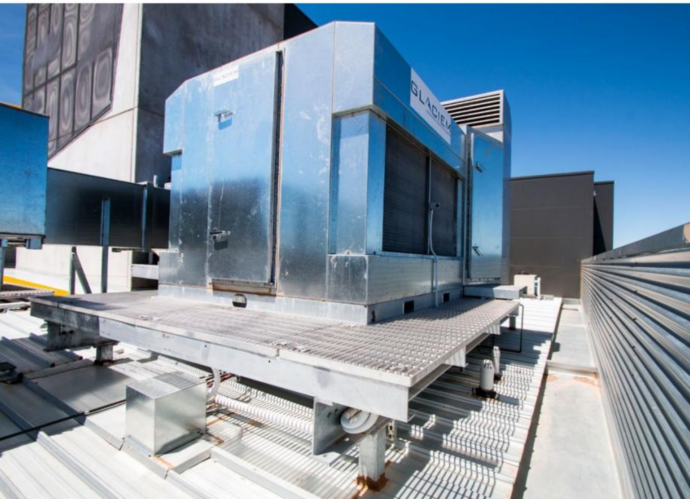
CO 2 condenser/gas cooler integrated with a Dew Point cooler.
