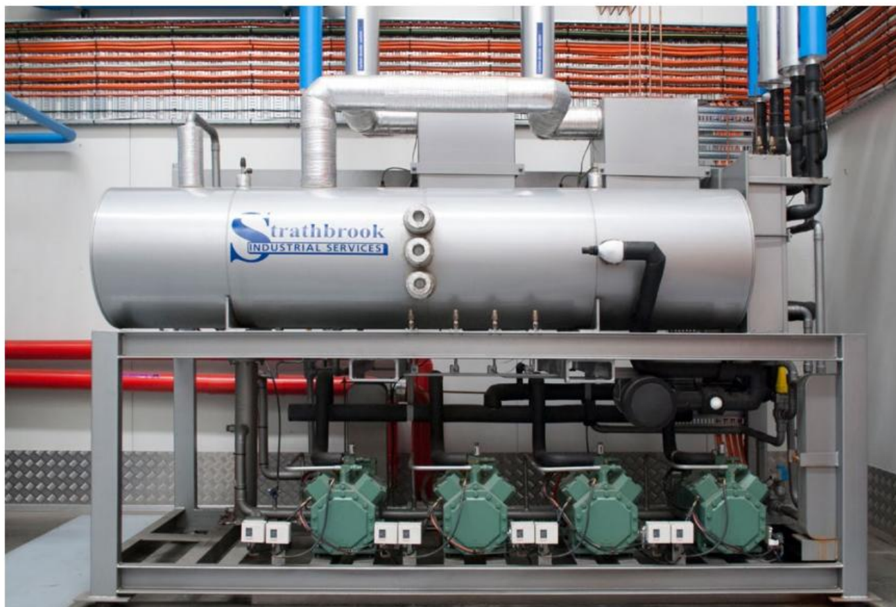
Low-stage CO 2 system for freezer room
