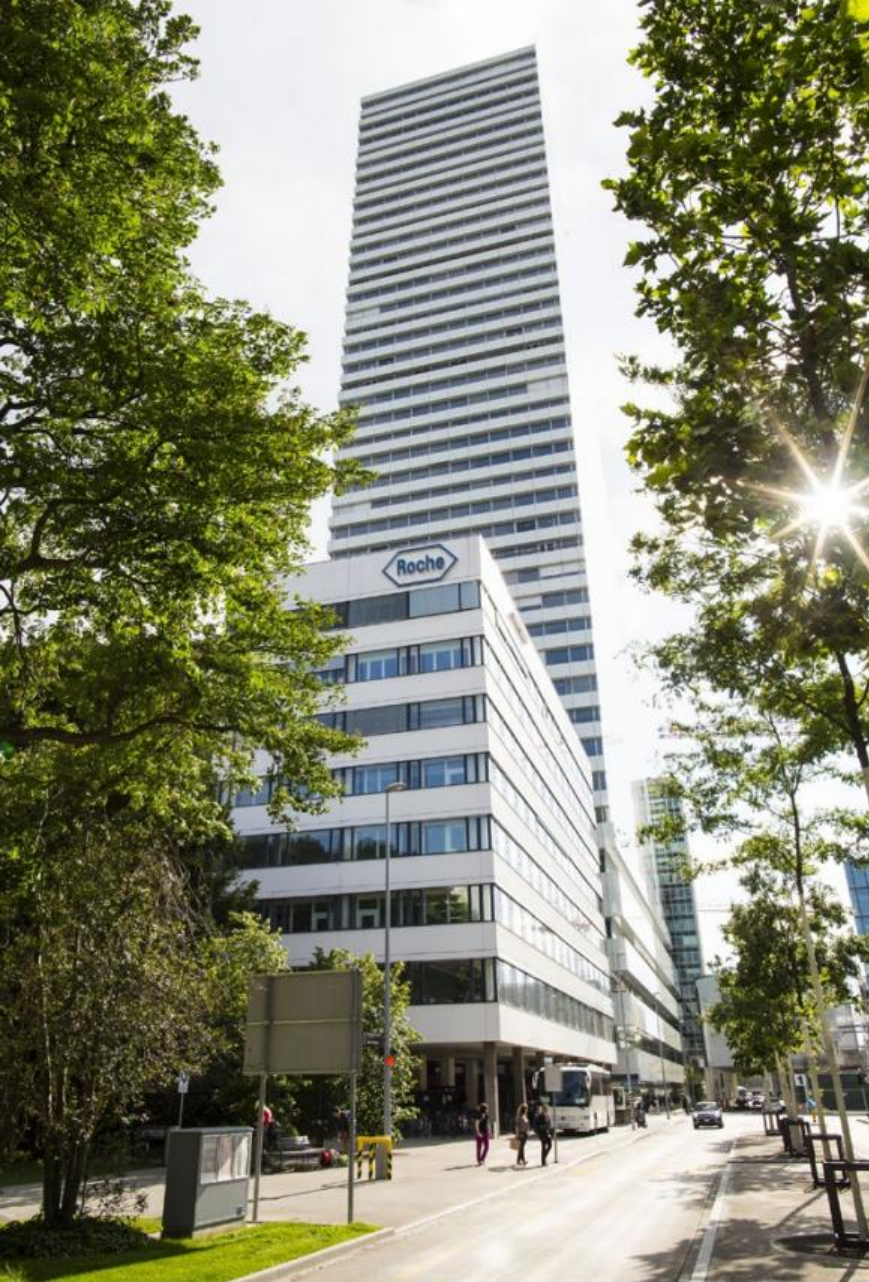
F. Hoffmann-La Roche headquarters in Basel, Switzerland.
