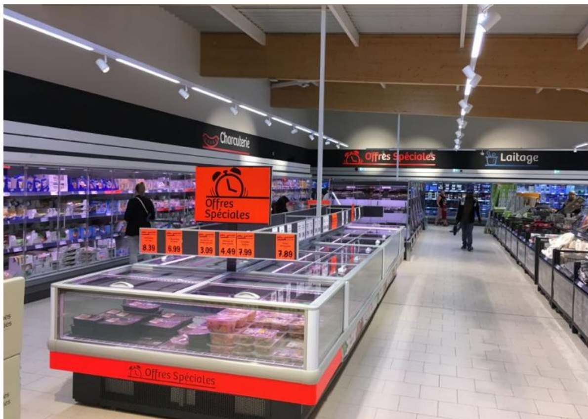
Propane cases in Lidl Valenton, the first Lidl France store to be 100% propane-based.
