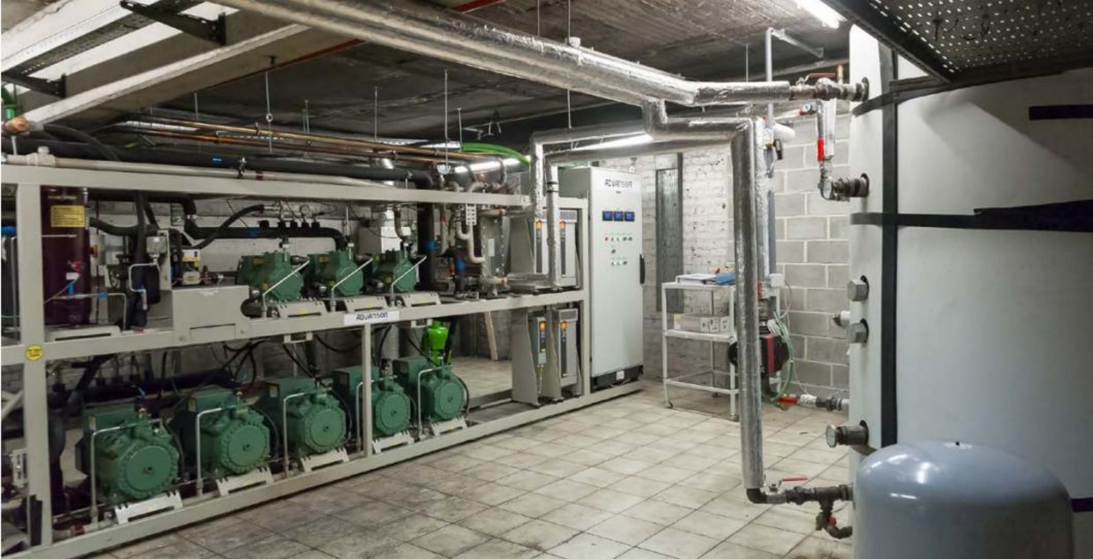
Heat reclaimed from the rack warms the greenhouse on the roof.
