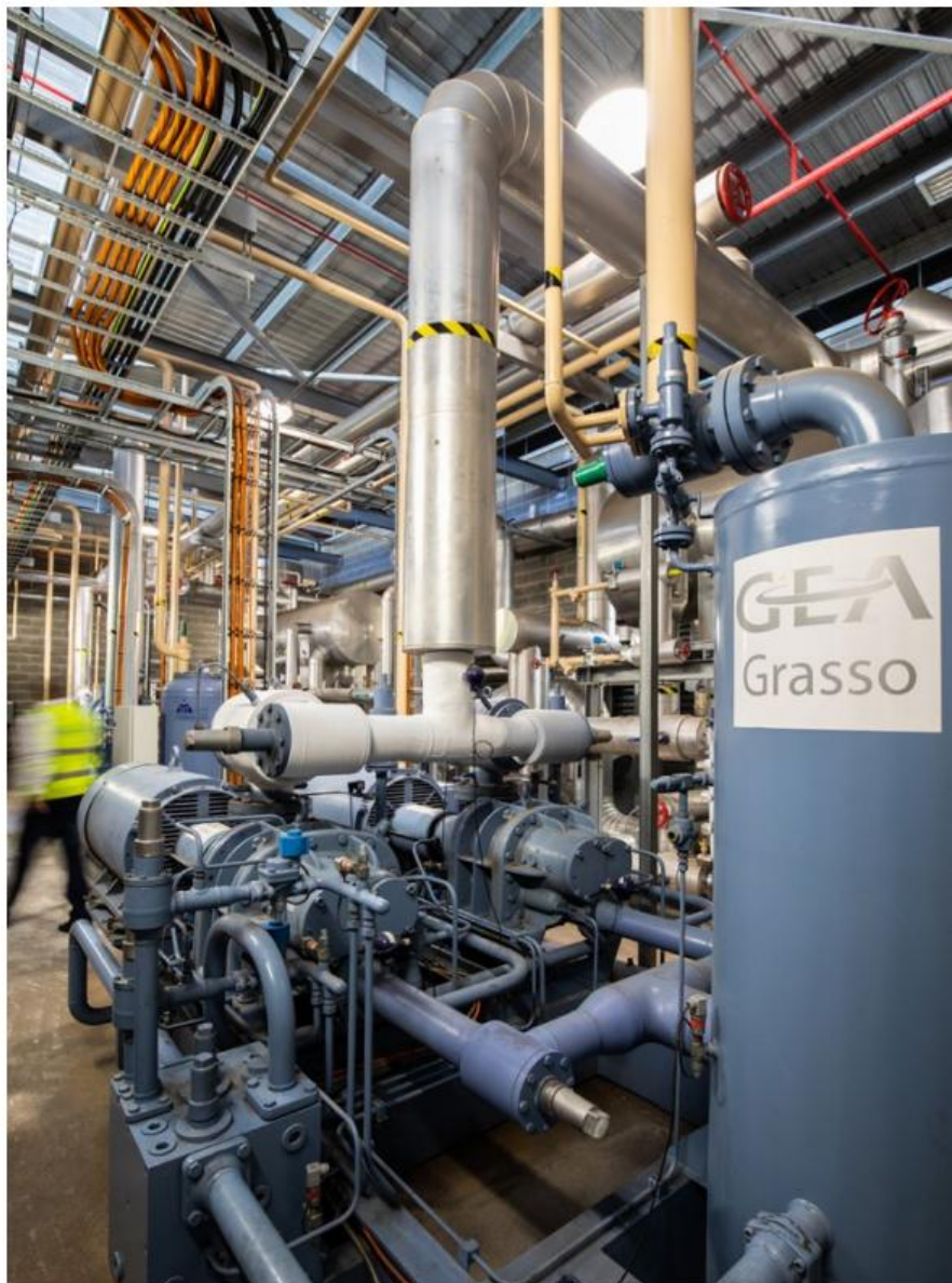
GEA Duo Pack compressor package for propylene glycol chilling duty.
