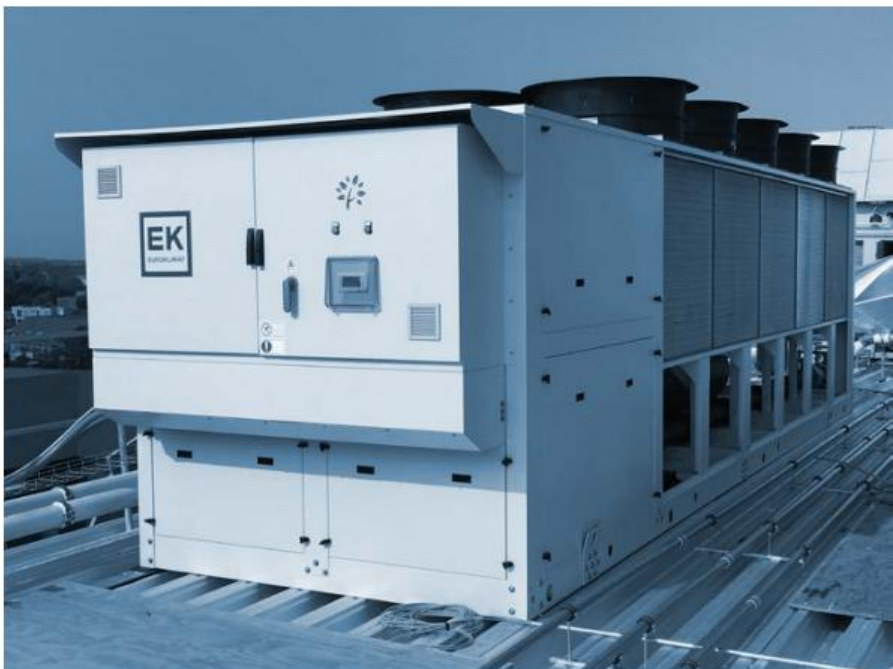
A Euroklimat propane chiller.
