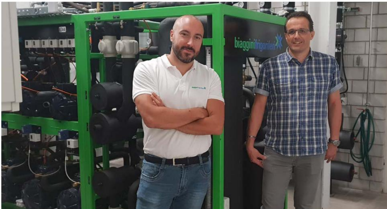
From left: Luca Rossi, Biaggini Frigoriferi, and Andrea Skory, Migros Ticino, with CO 2 compressor rack at Migros store in Riazzino, Switzerland
