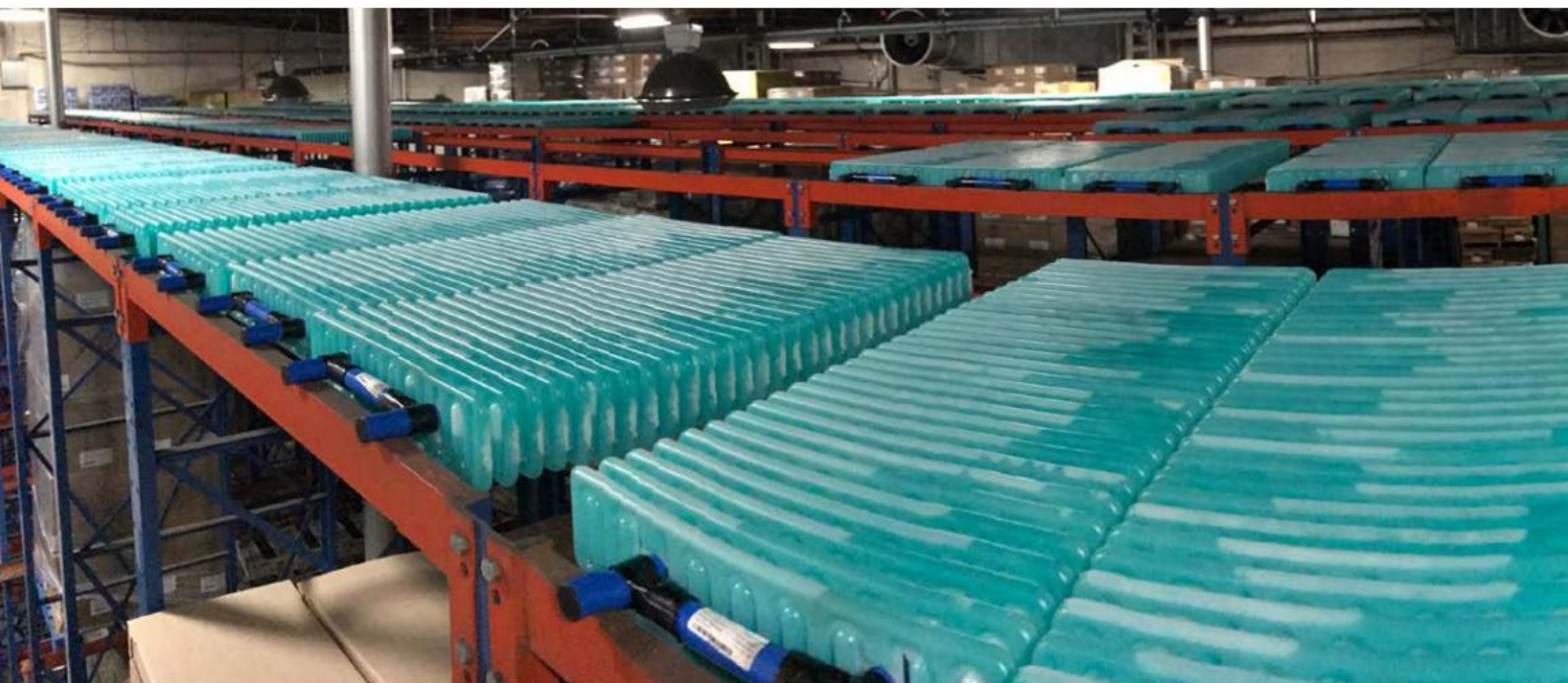
Viking Cold Solution's thermal storage cells at Dreisbach distribution center in Richmond, Calif.
