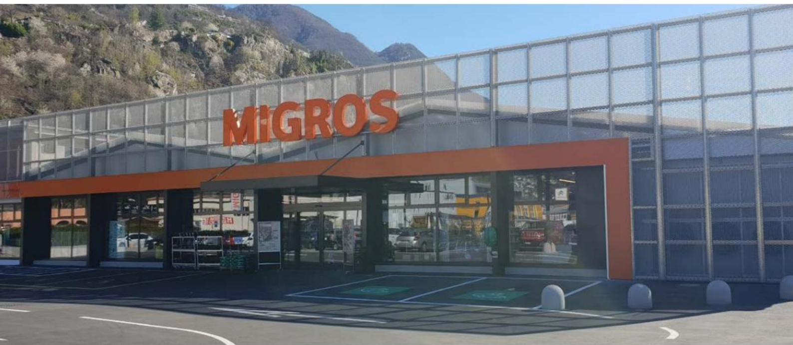
Migros store in Riazzino, Switzerland, with integrated CO 2 system
