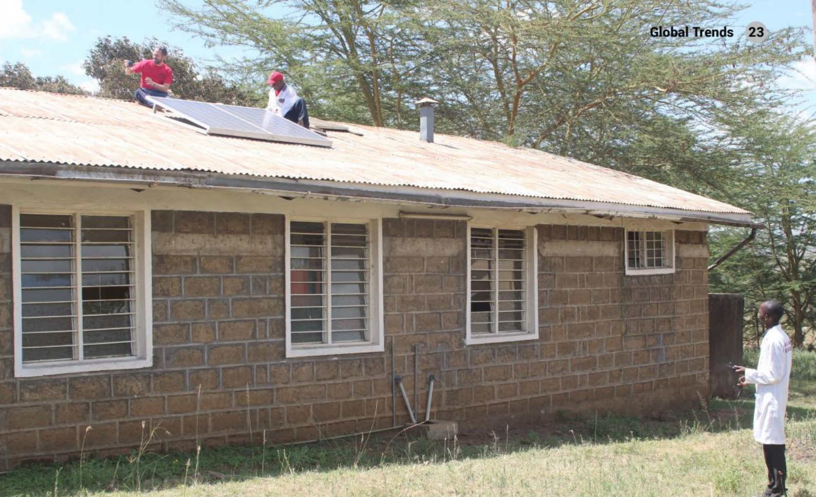
Installing a SolarChill fridge at the Olasiti Health Care Facility in Tanzania.
