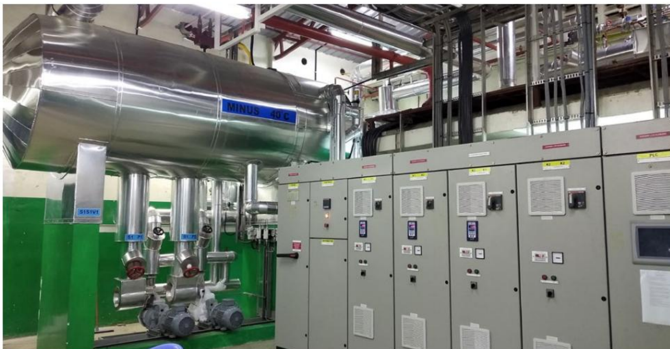
The system has a total ammonia charge of approximately 1,400kg (3,086.5lbs).
