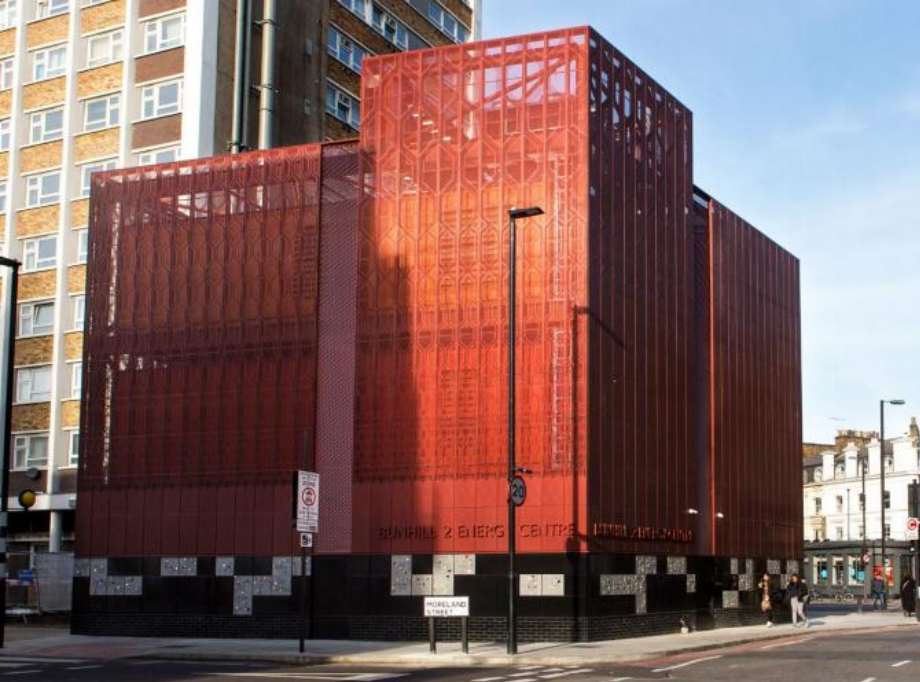
The Bunhill 2 Energy Centre
