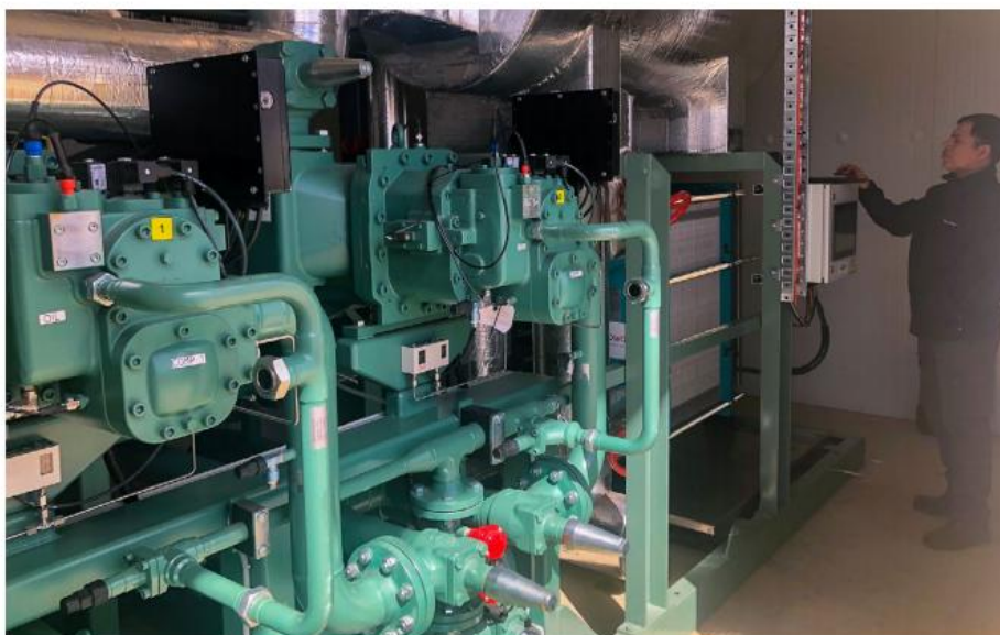
Bitzer's Green Point commissioning underway.
