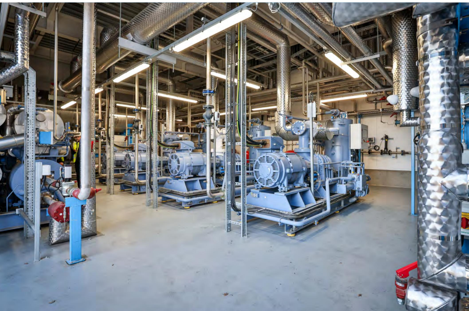
Engine room at Cranswick's prepared poultry facility in Hull, U.K., with four GEA screw compressors (right) and heat pump (left).
