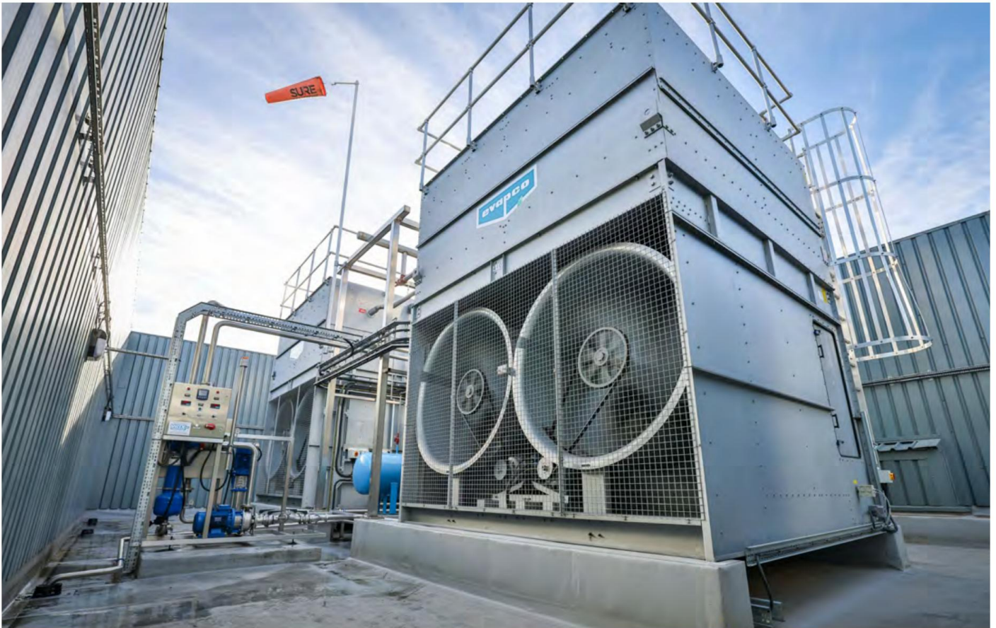
Evapco evaporative condensers on roof of Cranswick's prepared poultry facility, with ammonia receiver (light blue) and chemical-free water treatment system.
