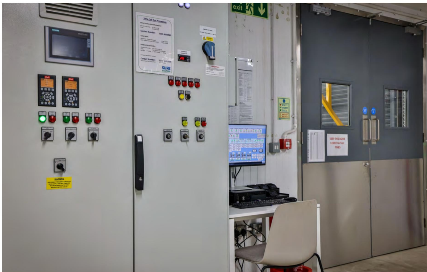
Computer (right) at Cranswick's prepared poultry facility that manages all switchgear, variable speed drives, leak detection panels, ventilation panels and other components, with ammonia leak-detection panel (middle) and ventilation panel (left).
