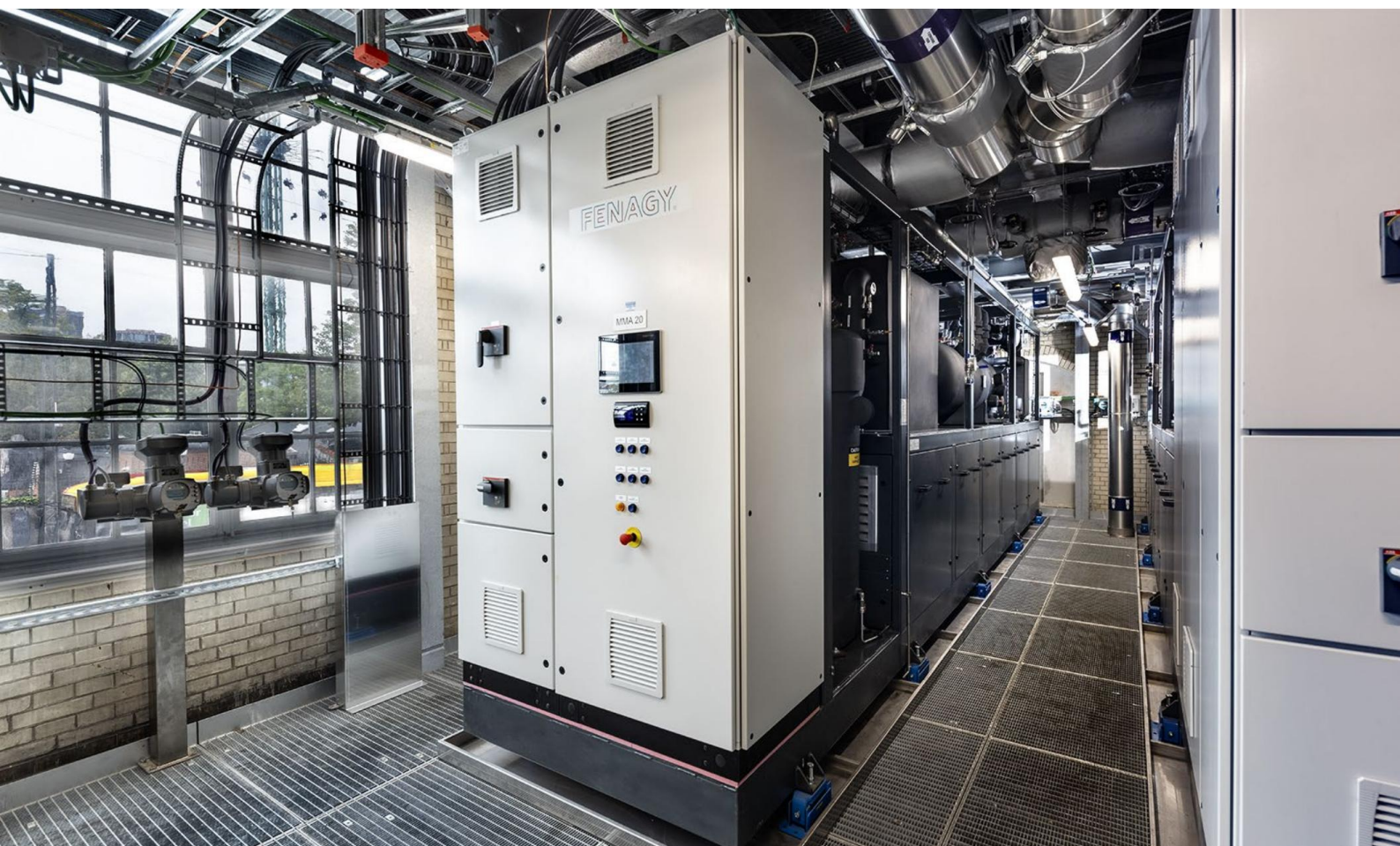
Two of the three Fenagy CO 2 heat pumps installed at the Tietgensgade facility with compressor panels and vibration feet. Photo credit: Fenagy
