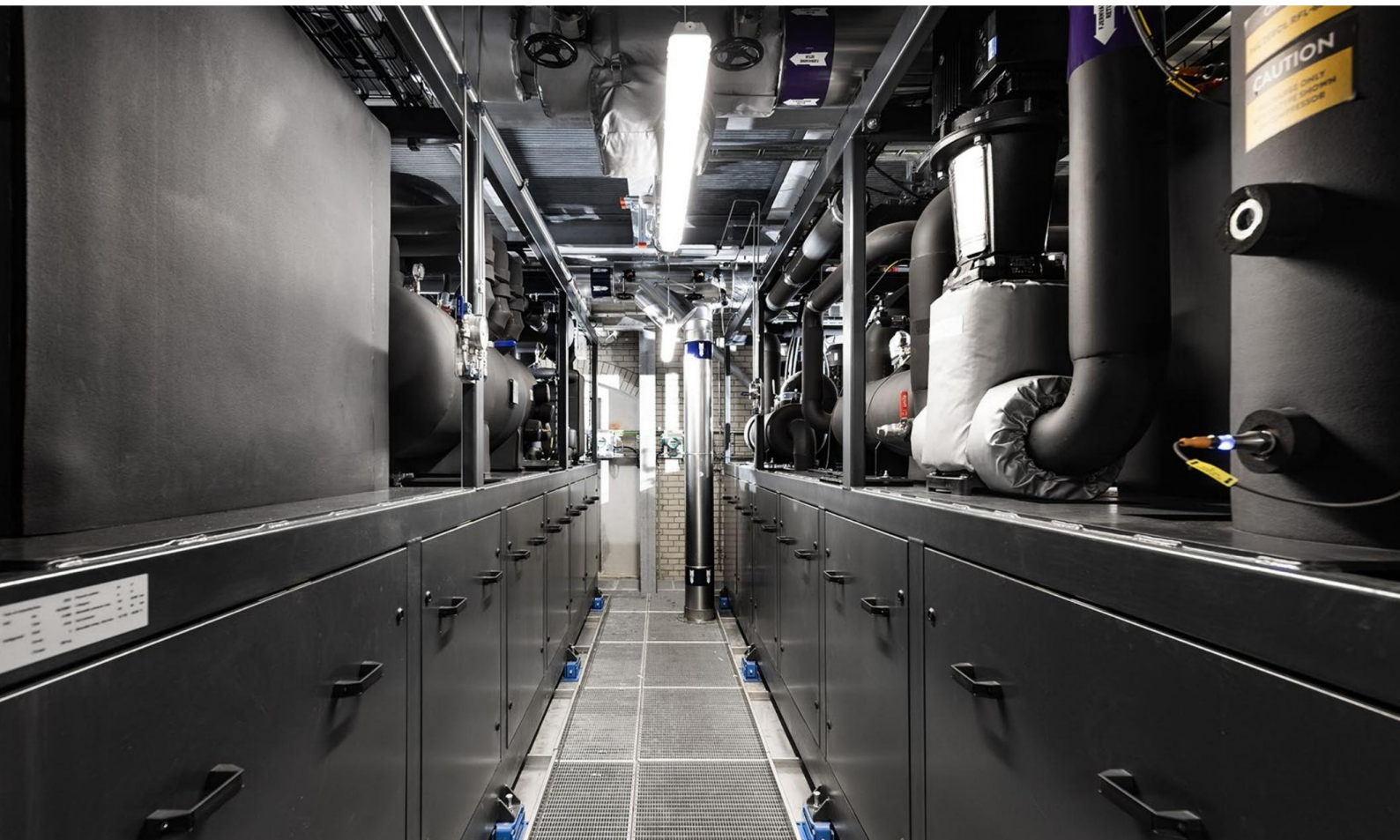
The three CO 2 heat pumps from Fenagy provide 5.2MW of heating capacity and 3.6MW of cooling capacity. Photo credit: Fenagy
