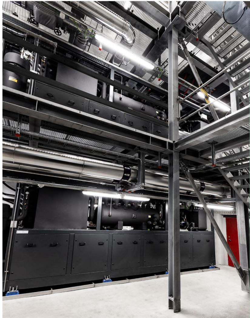
To get around space constraints, a mezzanine level was installed so the heat pumps could be stacked on top of each other. Photo credit: Fenagy
