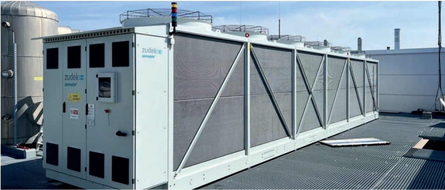
Zudek's Airmatik ammonia chiller being installed at a data center. Photo credit: Zudek.
