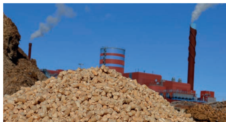
Right: Wooden pellets produced at the Falu Energi & Vatten CHP facility. Photo credit: Falu Energi & Vatten.
