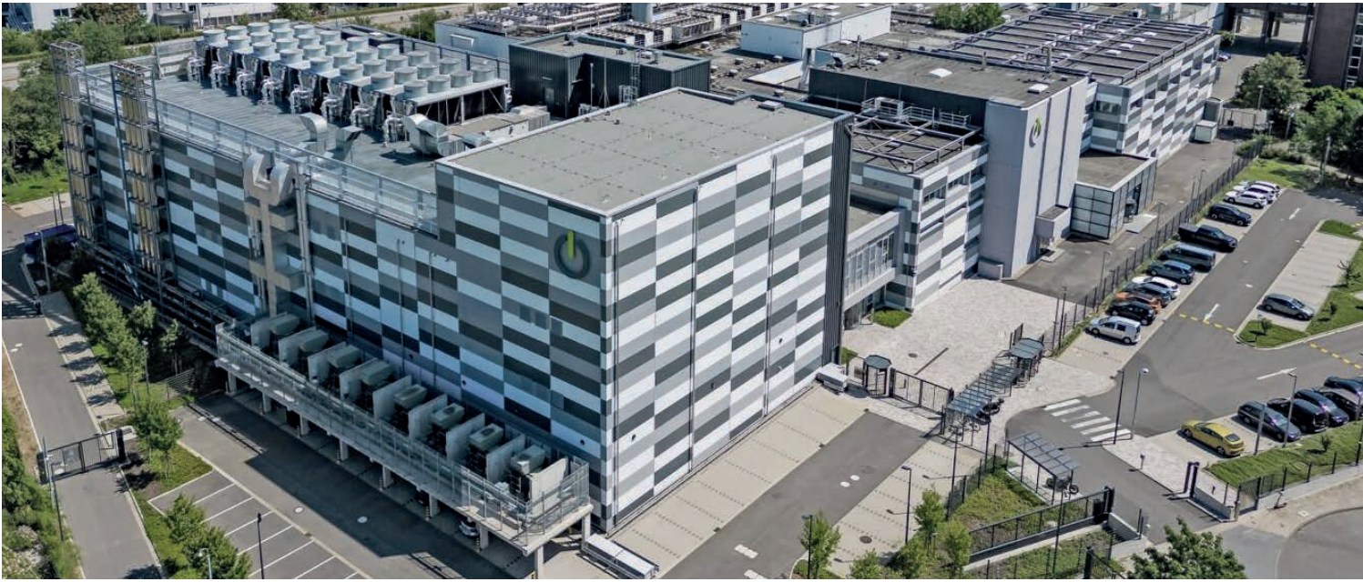
Jaeggi's HTK hybrid dry coolers installed on the roof of Global Switch's Frankfurt North data center in Frankfurt, Germany. Photo credit: Mercury.
