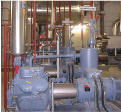
image 7: GEA Grasso 65HP compressors with variable-speed drive motors for optimised operation under partial load
