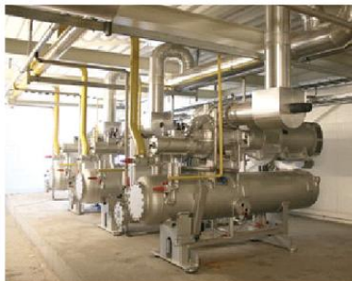
image 6: Three SAB193L compressors produce the refrigeration at Zellik
