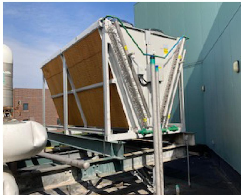
CO 2 gas cooler at Santander Arena; Nationwide Arena will install the same model in 2023.
