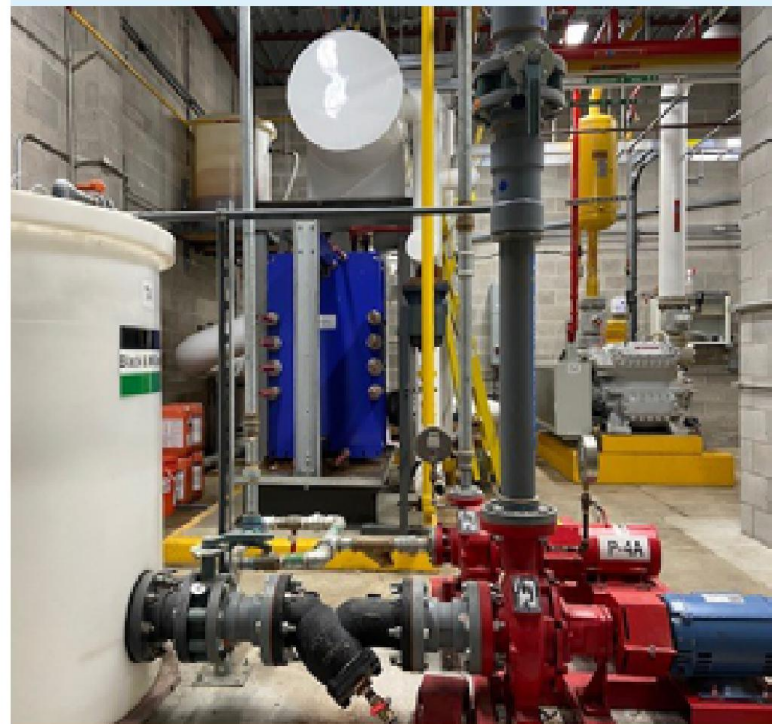
At left: white evaporative condenser water tank; at middle, rear: blue plate-and-frame heat exchanger, Pickering ice arena.
