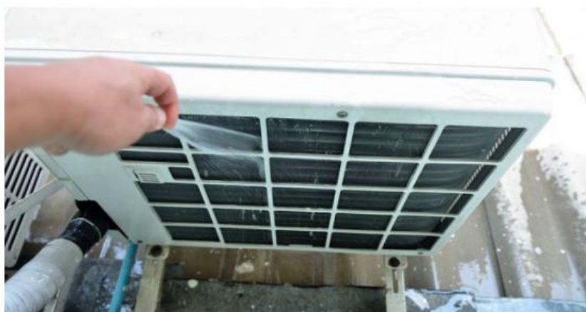
Below: Cleaning of dirty equipment
