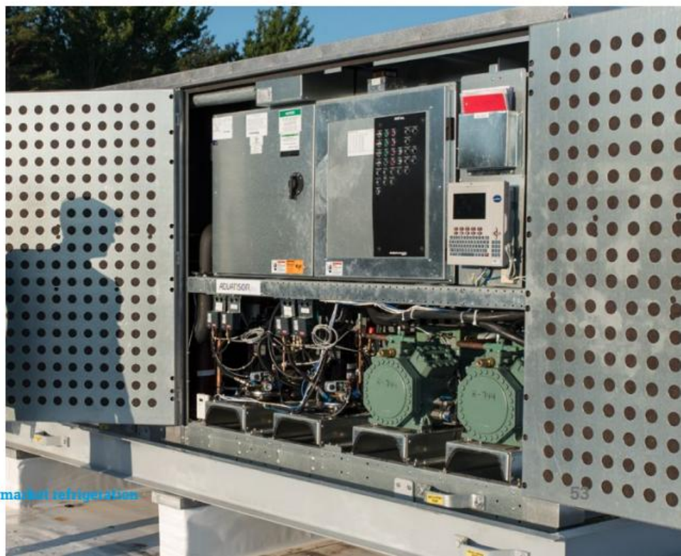
Below: CO 2 transcritical rack used at an ALDI US store in New York
